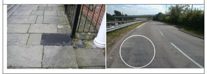
**Condition 4 "Functionally impaired" =** Signs of defects i.e. cracking, fretting, potholes, subsidence all defects above intervention levels – **AMBER**
