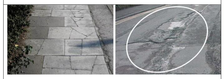
**Condition 5 "Structurally impaired" =** As grade 4 together with major signs of defects to structural layers or compromised sub base visible – **RED**
