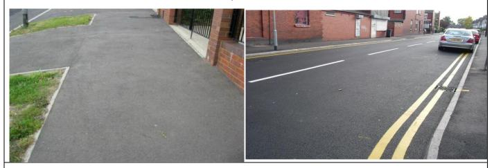
**Condition 2 "Signs of surface wear" =** Good condition – may comprise modular construction with elements of different colour/age/material, Faded bituminous materials (especially coloured bituminous), Graffiti or Spray paint etc. – **BLUE**
